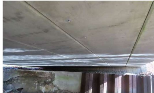
Photo 2: Typical underside, looking east.
