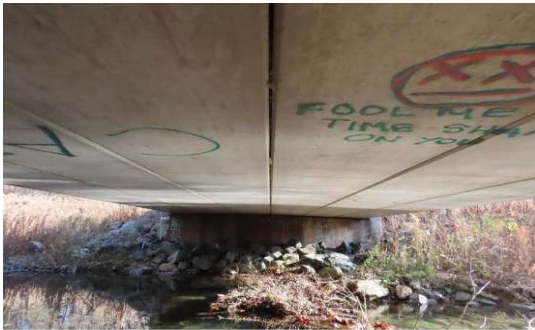
Photo 2: Typical underside, looking east.
