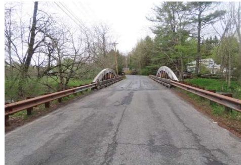
1: General topside, looking north.
