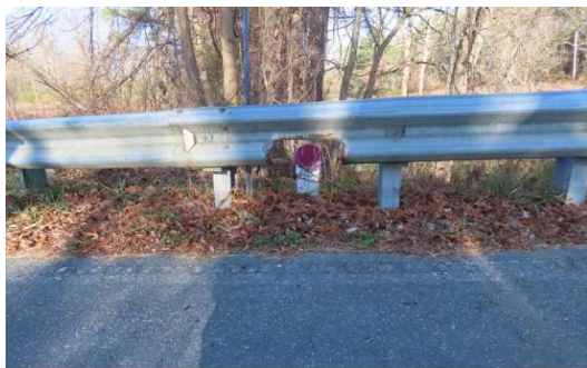
Photo 6: Cut panel in the northwest transition.
