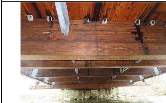
2: General underside, looking south.
