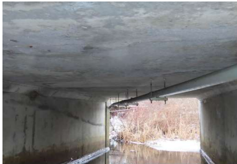
2: General underside, looking east.
